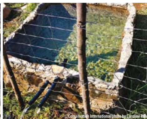
Above - This collection chamber receives water from the pipes at the back of the tank and the overflow at the front is available for collection as needed.
